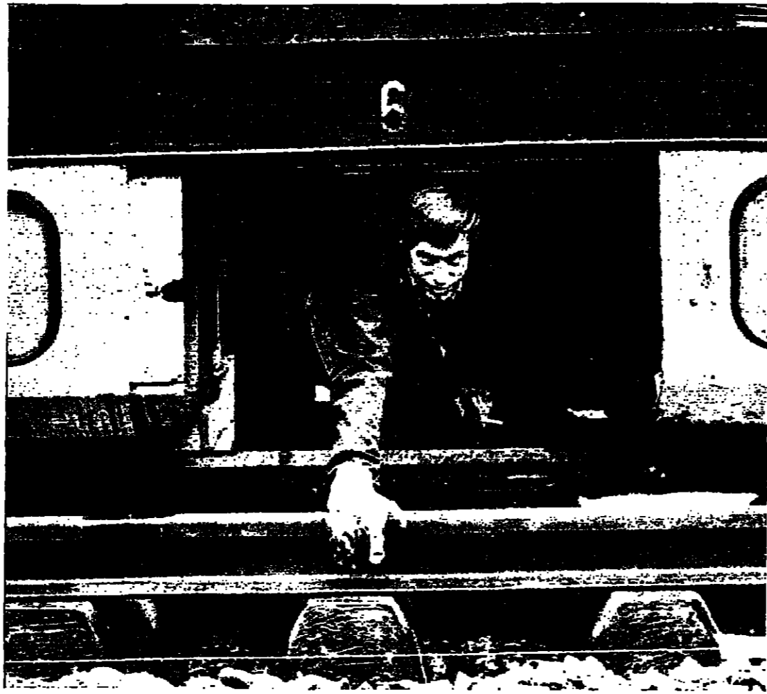
STRONG MAN -- West Germany's track-laying trains are the modernistic way of building railways. This equipment can lay a section of 2.5 kms in one day. The old track is raised automatically, and the sleepers removed. The caterpillar track equipment then lays the 120-metre-long welded track complete with new sleepers, carrying out the work of about 1,500 strong men. The man in the picture, working in an air-conditioned cabin, is loosening the bolts that fix the rails to the sleepers, but every tenth bolt is left in place for safety's sake.
